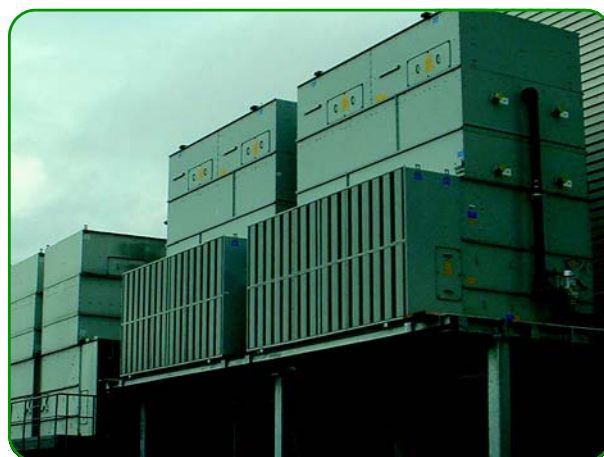
Unit with Intake and Discharge Sound Attenuation
