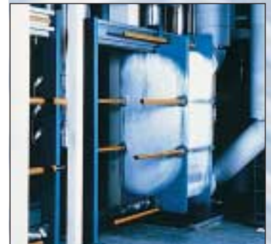
One of three ammonia glycol evaporators in stainless steel installed in a brewery to replace shell-and-tube heat exchangers of carbon steel in a brewery.
