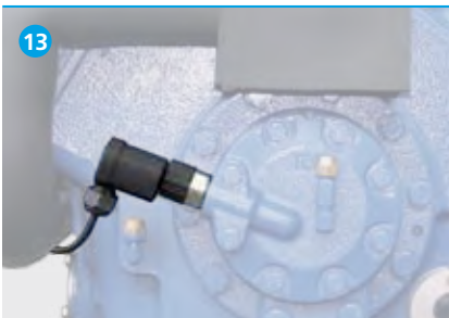
Oil differential pressure sensor
