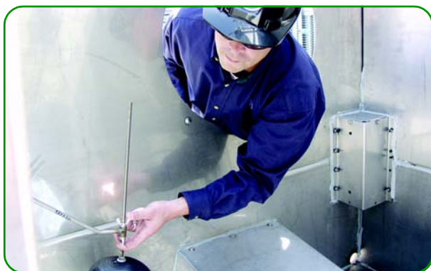
The water level control is easily reached from the access door.
