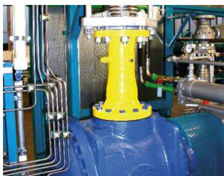
Gas Turbine Installation
